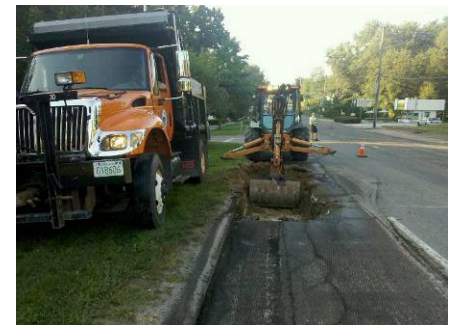
DW Repair Prior to Paving
