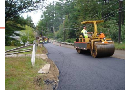
Paving Binder on Reclaimed Base.
