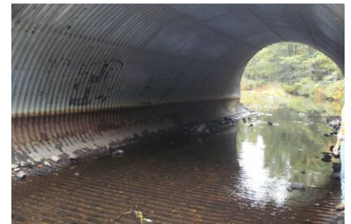
Inside pipe arch – note corrosion at spring line.
