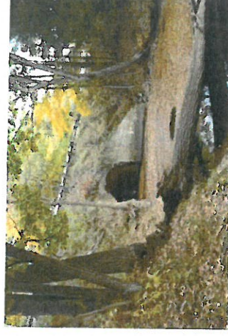
US 3 bridge, downstream side.
