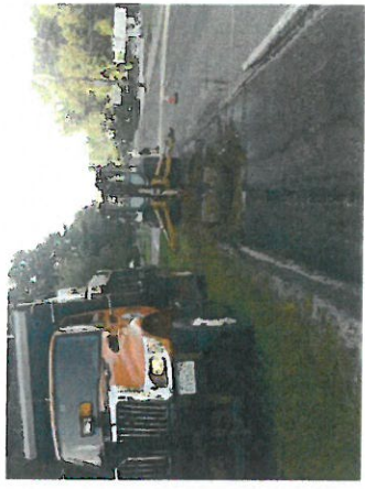
DW Pavement Grinding
