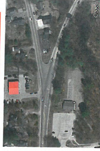
Aerial View of Wire Road/DW Highway Intersection.
