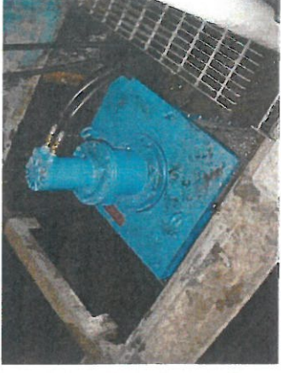
Original Raw Wastewater Solids Grinder 1970
