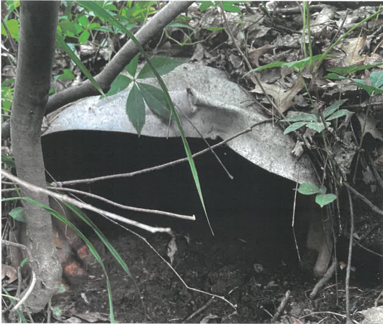
West end of culvert.
