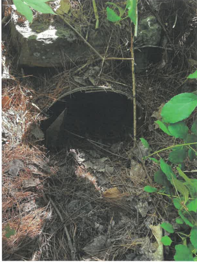
North end of culvert.
