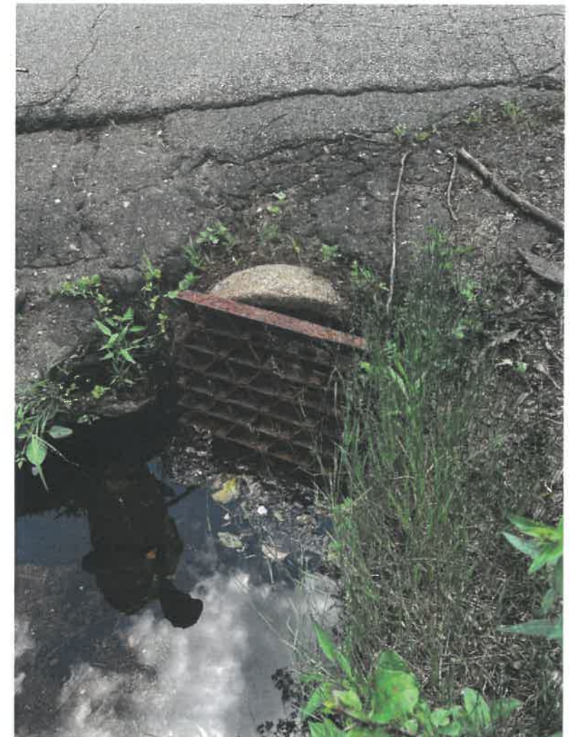
North end of culvert.
