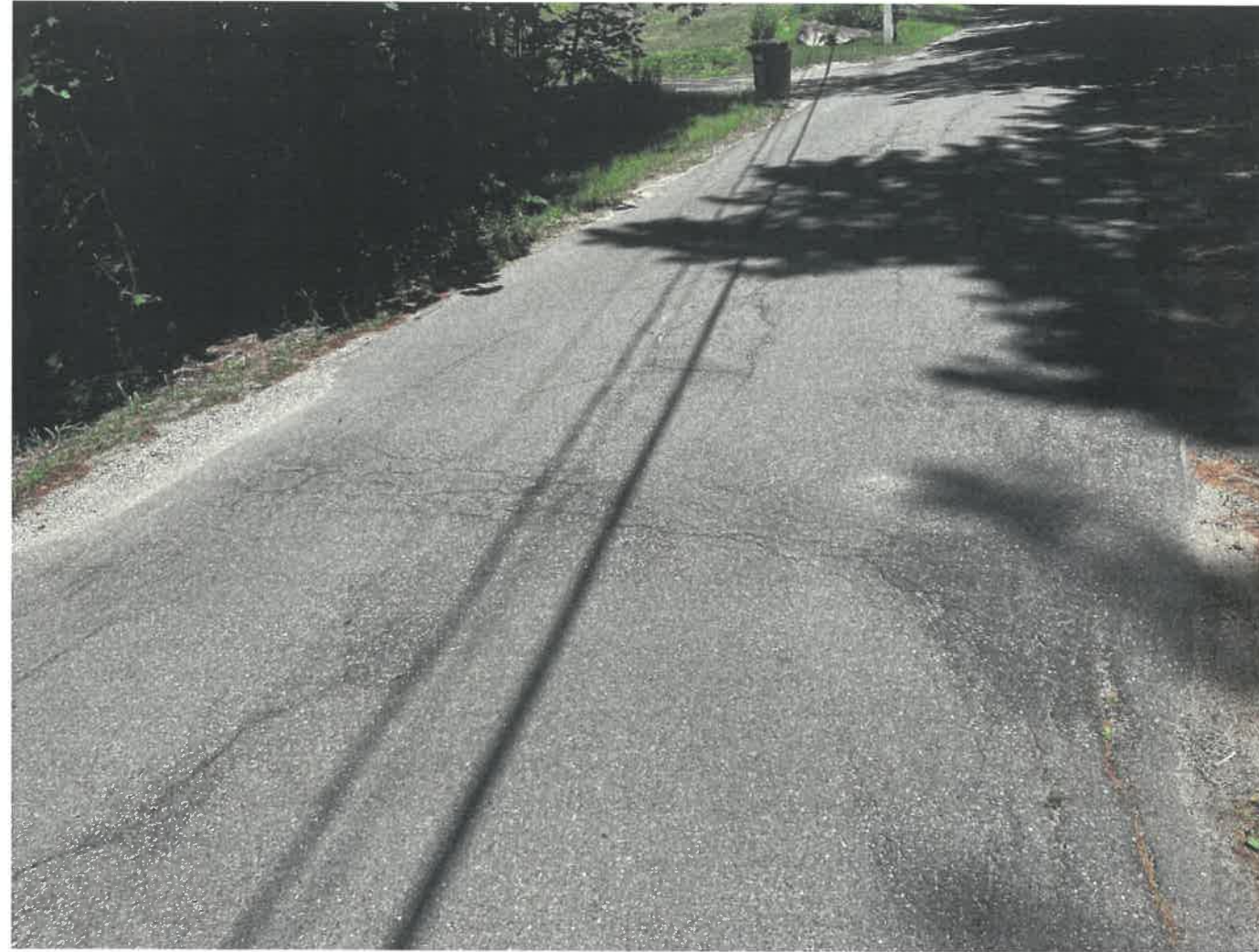
Top of culvert on Thornton Road West facing east.
