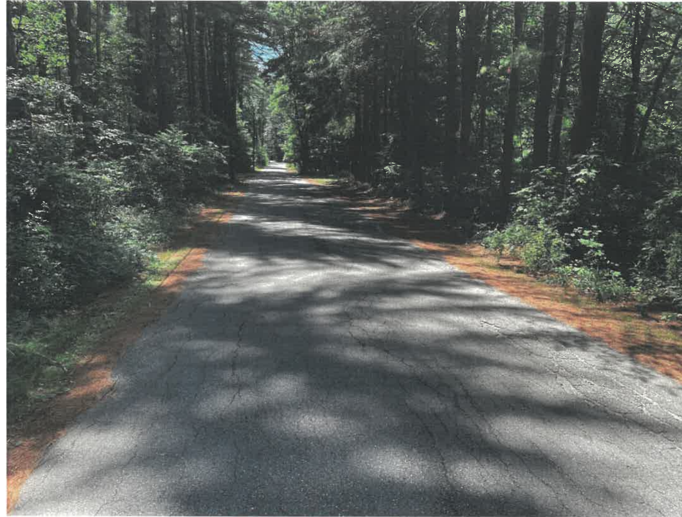
Top of culvert on Thornton Road West facing west.
