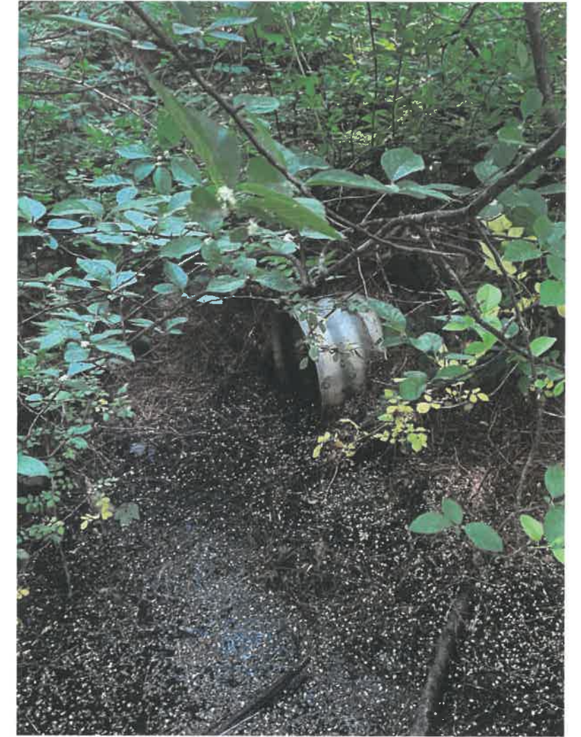
South end of culvert.
