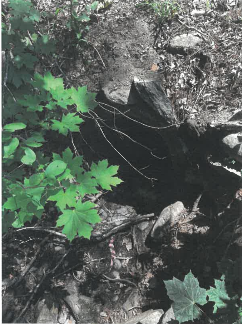
North end of culvert.
