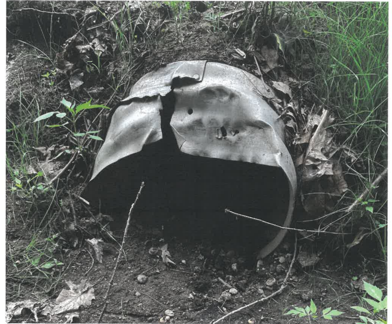
East end of culvert.
