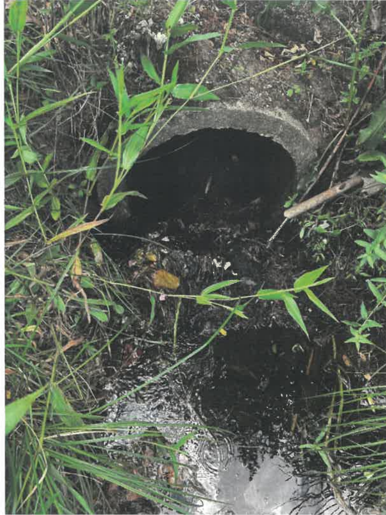
South end of culvert.
