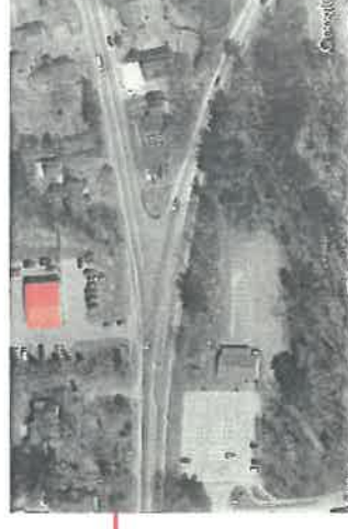
Aerial View of Wire Road/DW Highway Intersection.
