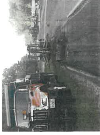
DW Pavement Grinding
