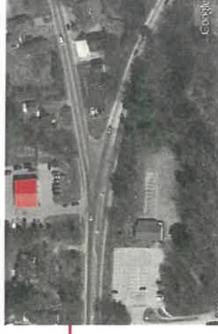
Aerial View of Wire Road/DW Highway Intersection.
