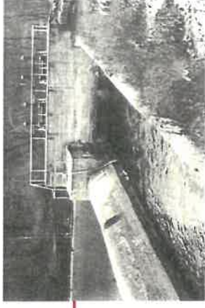
Historic view of sluiceway and headgate
