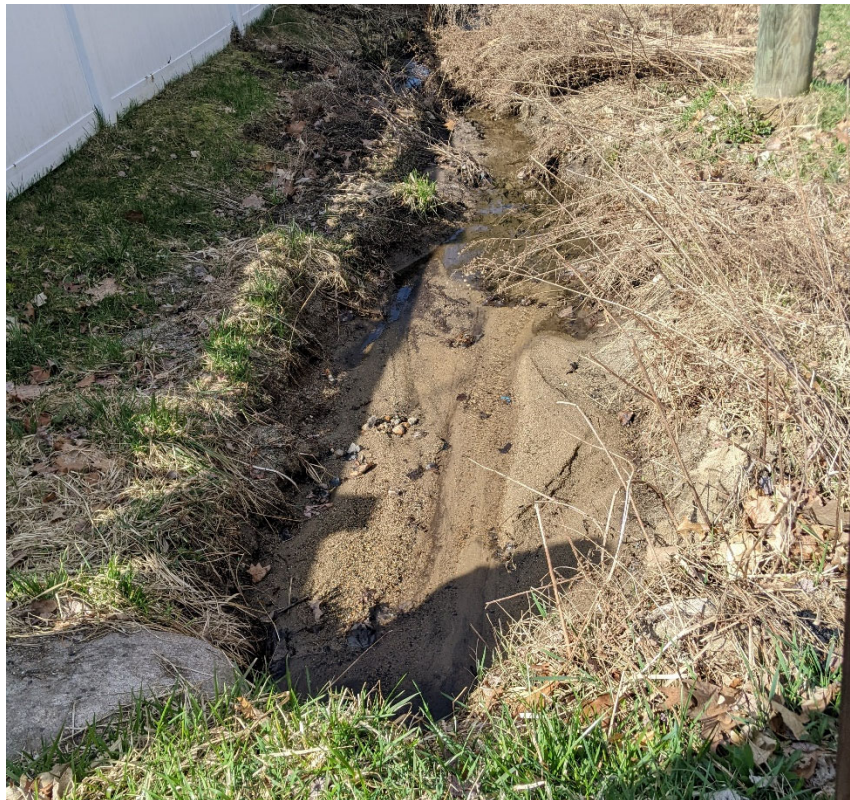
Photo 1. Silt-filled roadside swale along Carter Road. Swale accepts significant load from unpaved Rennie road.
