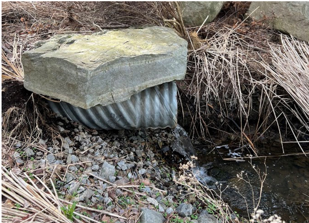
Photo 2. Primary outfall to Baboosic Lake at end of Carter Road
