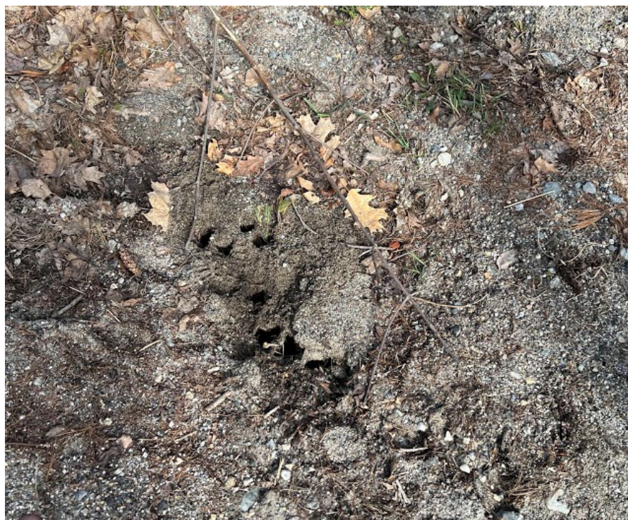
Photo 8. Former BMP Overflow catch basin at Carter & Arnold covered by 2" sediment (note: Carter is paved; Arnold is unpaved).
