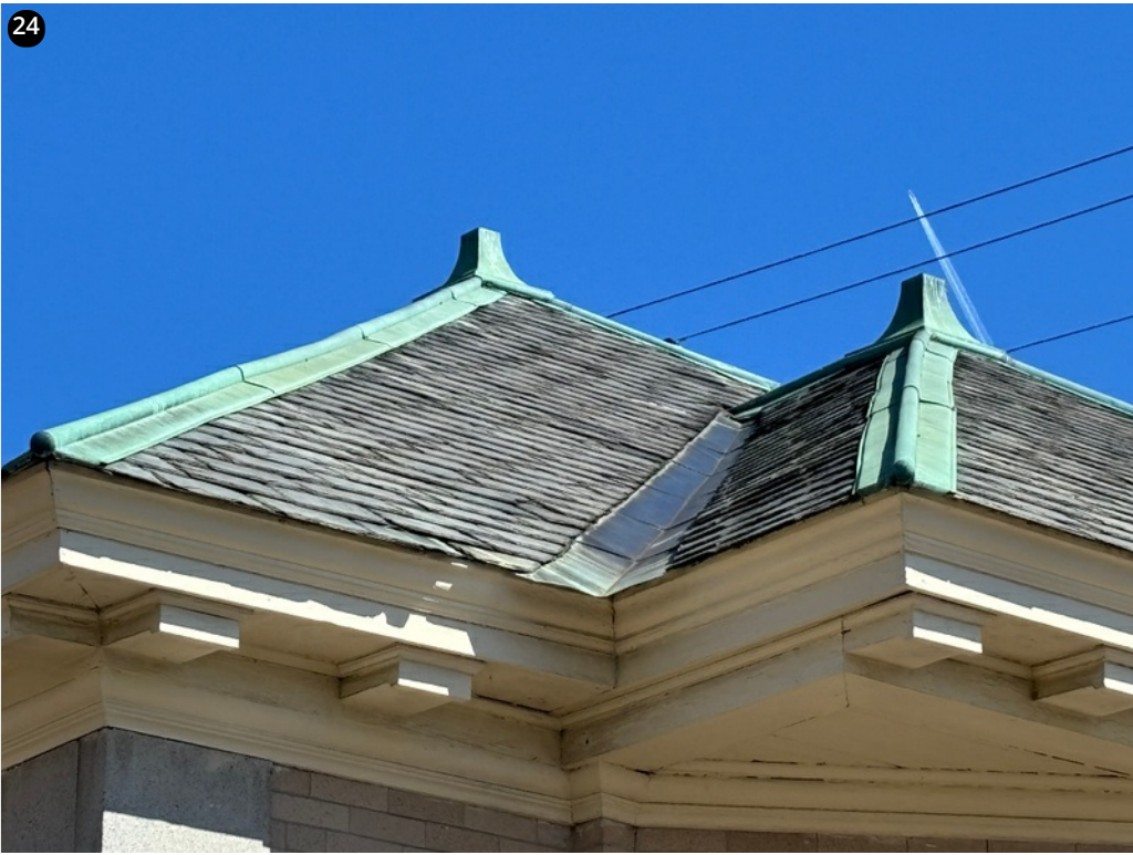
Photo showing South facing slate roof section.
